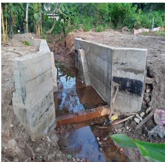
Photo 25 : Renovation of Malwarusha Canal
