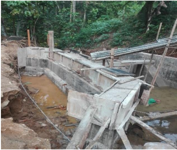
Photo 27 : Construction of Jayavindagama Murutagaha Pela Anicut
