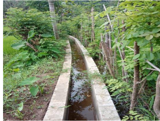
Photo 39 : Renovation of Bulat Val Kandura Canal, Kandy District
